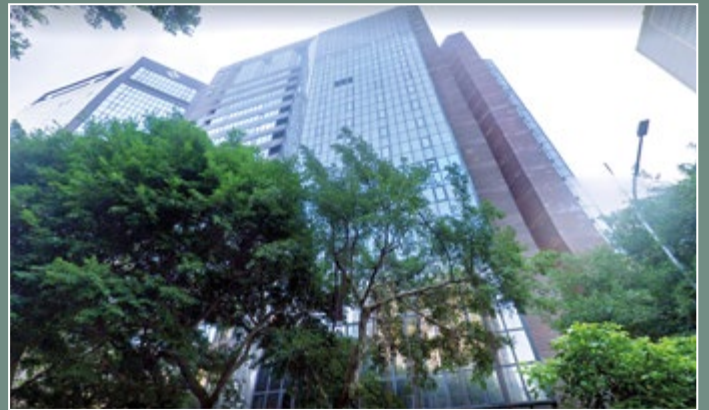
Tapei Operations Center Operations Center
