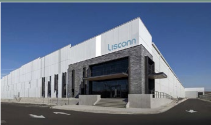
Tijuana Manufacturing Manufacturing Facility
